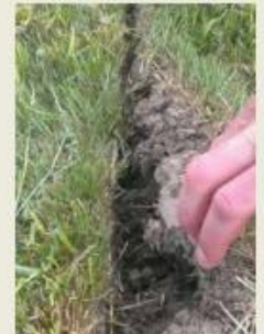
Targeted depositing of the slurry under the turf
